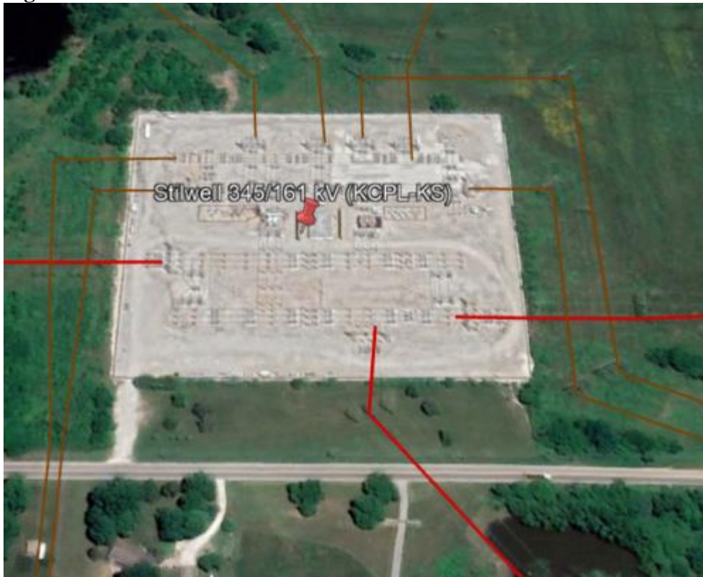
Figure 28 – Stilwell 345 kV substation
